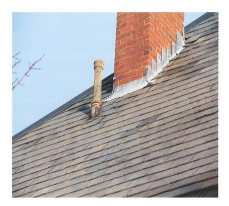
The vent pipe in the photo has an old lead boot on it that has been covered in tar and still leaks.
