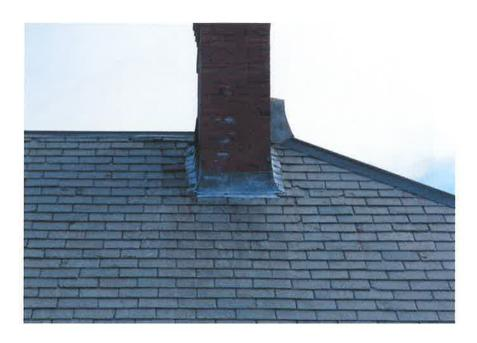
The chimney seen in this photo is incorrectly flashed and the pan above the chimney is a rotted piece of steel. There isn't any flashing in the roof and the chimney leaks.
